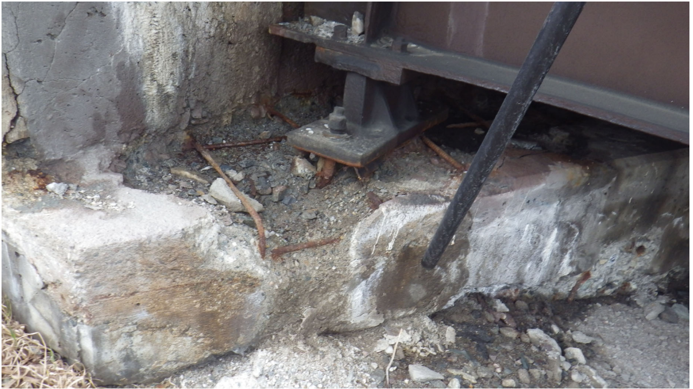
Picture 10: Abutment deterioration at bearing location
