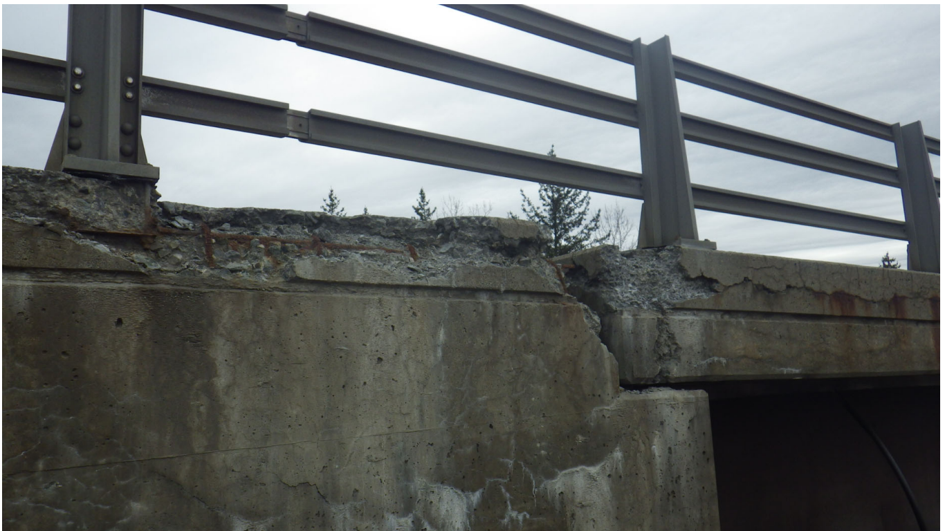
Picture 13: Curb Deterioration (note cracking and efflorescence on wingwall)
