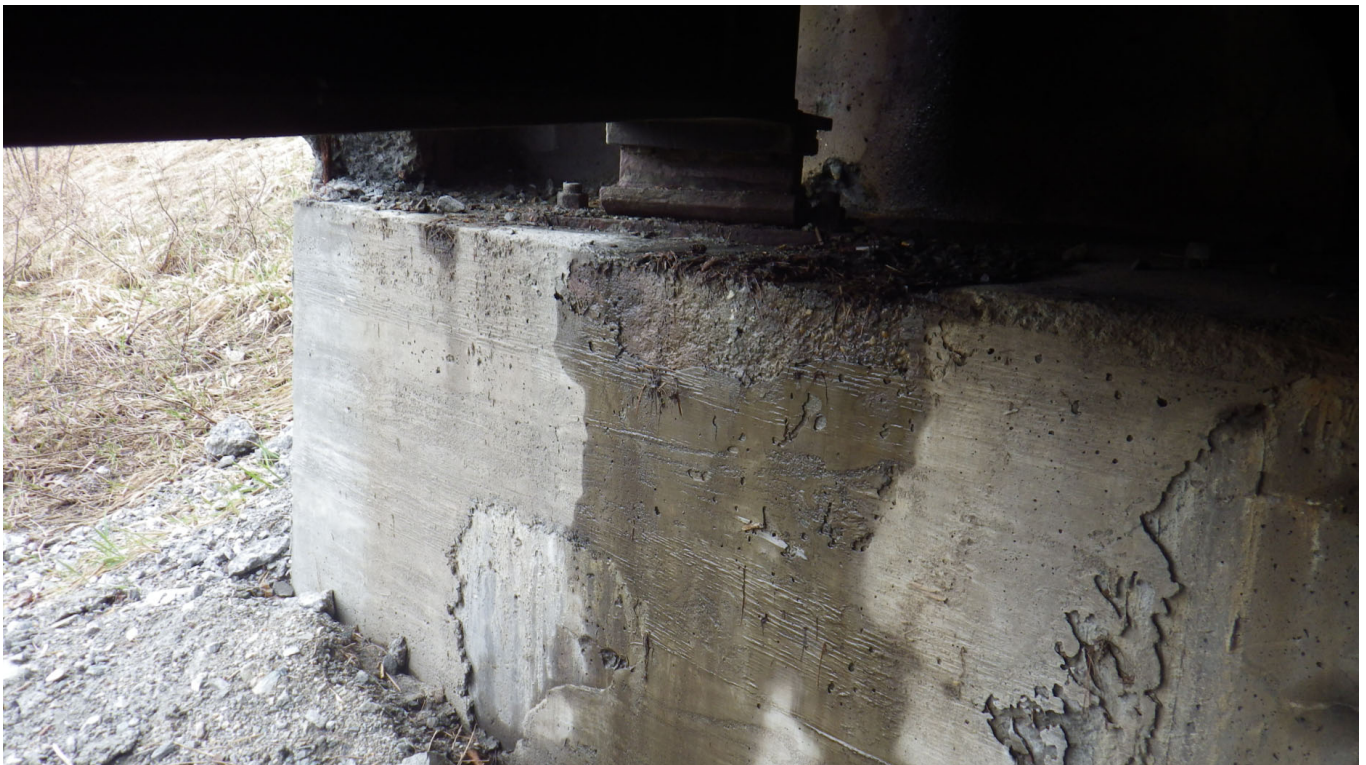
Picture 11: Water infiltration on abutment
