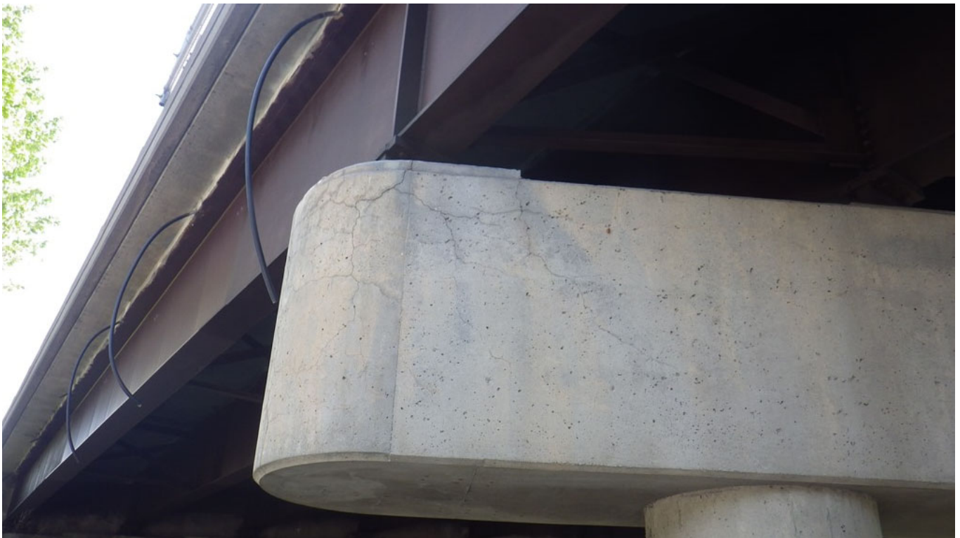
Picture 2: Cracking at pier cap nose
