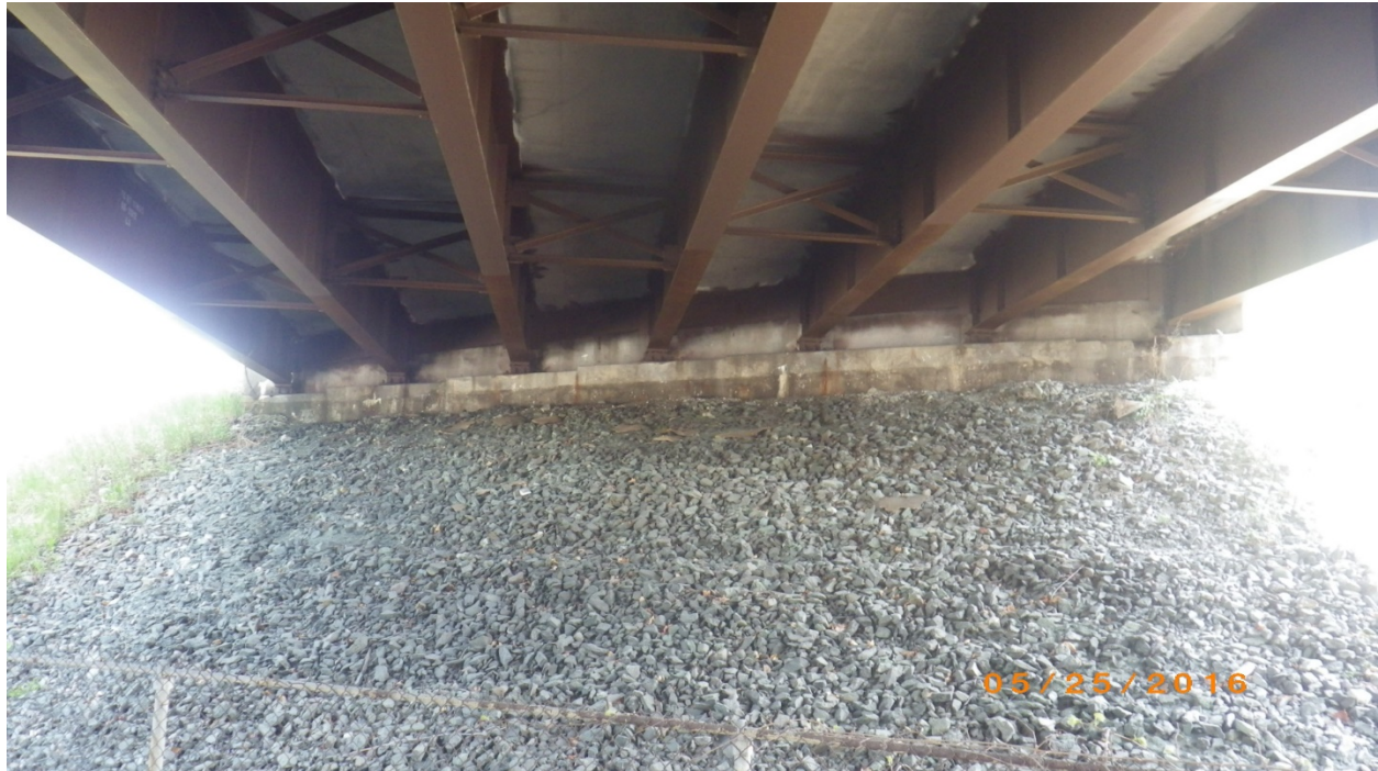
Figure 3.1: Stone fill armoring at bridge abutment. [Inspection photo dated 2016]
