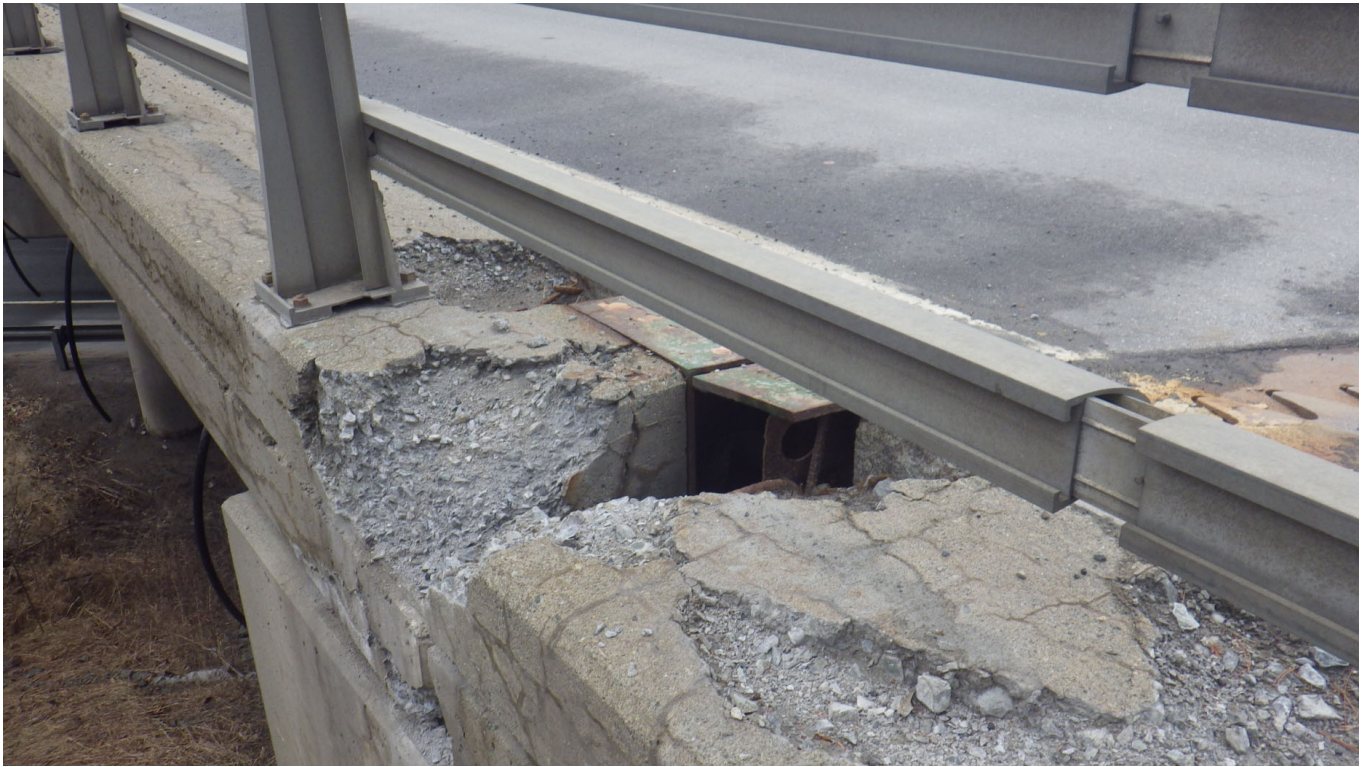
Picture 12: Curb cracking and deterioration
