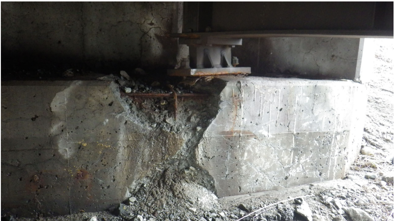
Picture 8: Abutment deterioration at bearing location
