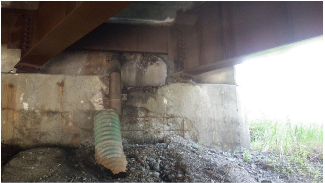
Picture 5: Abutment Deterioration
