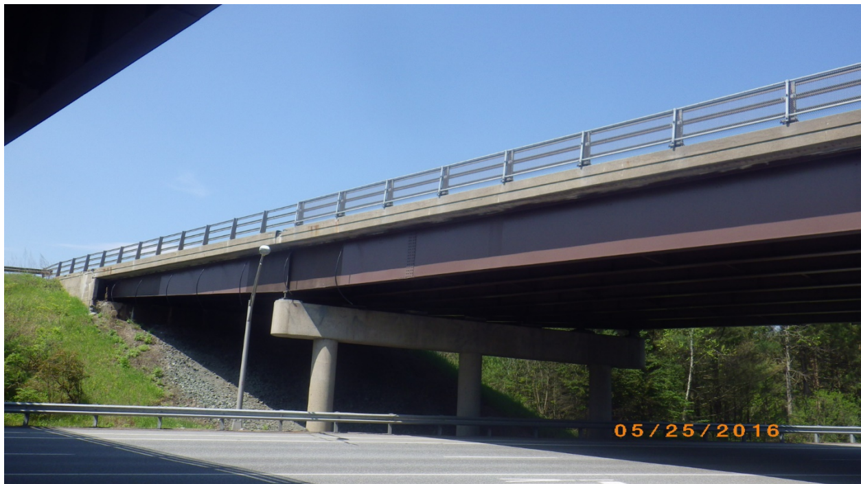
Figure 3.2: Facing I-91 Southbound south abutment; note limited overhead clearance for drilling operations under existing bridge. [Inspection photo dated 2016]
