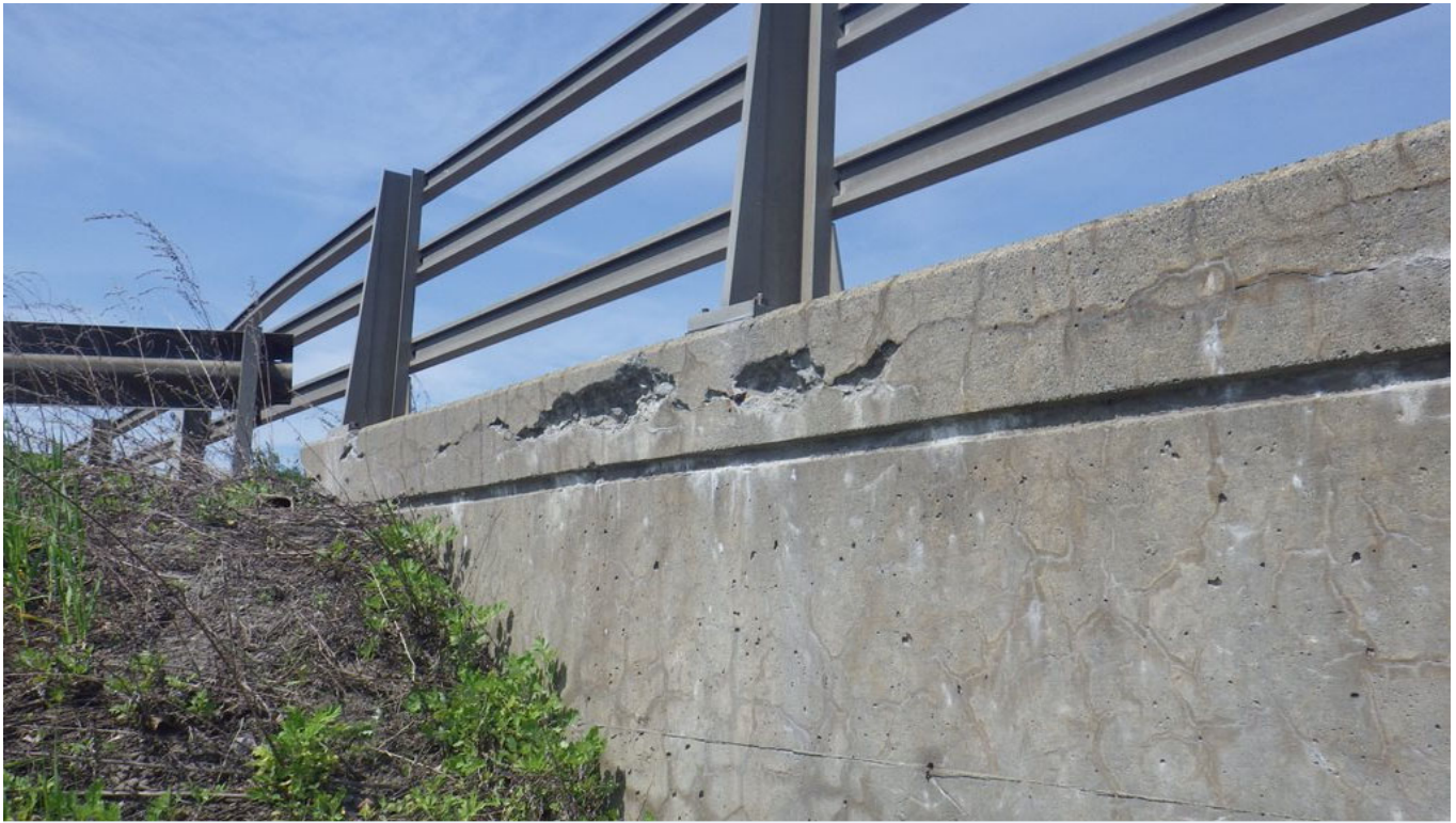
Picture 7: Wingwall cracking and curb deterioration
