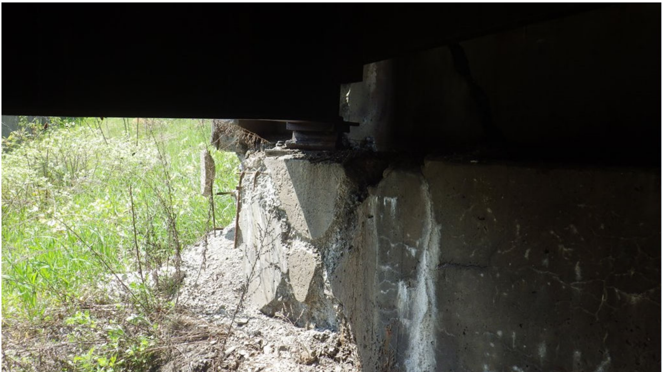
Picture 6: Abutment Deterioration
