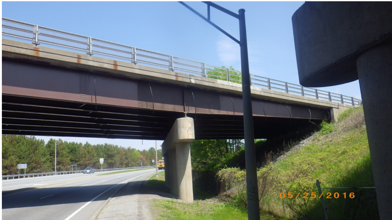
Figure 3.3: Facing I-91 Southbound north abutment; note limited overhead clearance for drilling operations under existing bridge deck. [Inspection photo dated 2016]
