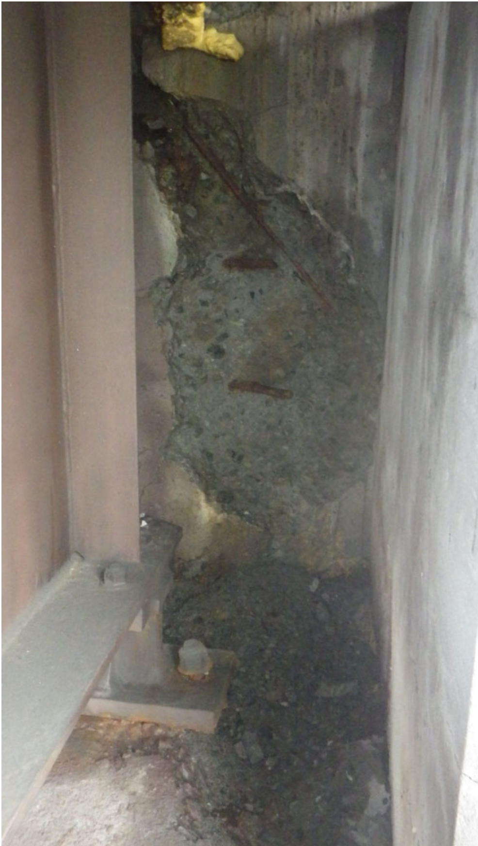
Picture 9: Poor backwall condition
